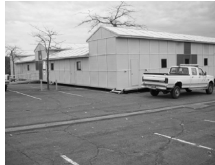
View from the Parking Lot
